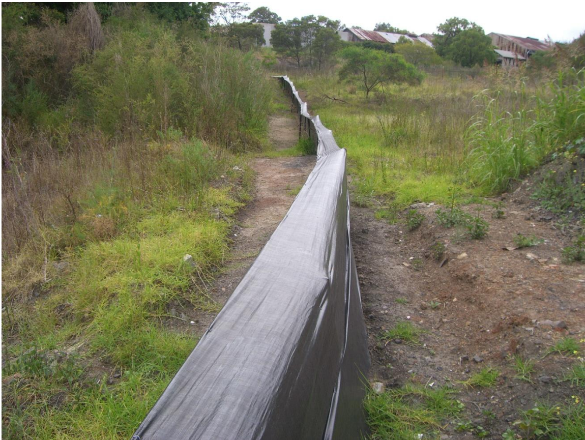
Figure 2 Frog habitat protection fencing near Coxs Creek
