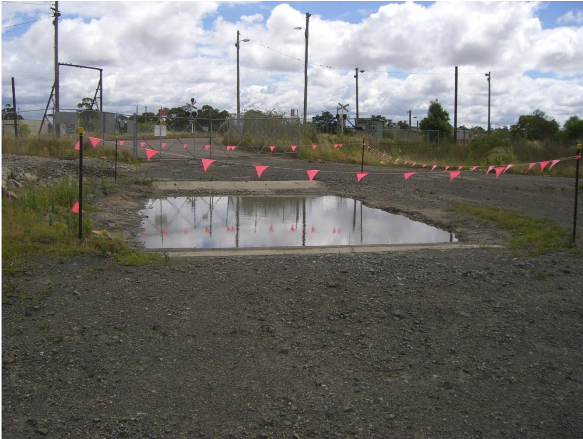
Figure 3 Wheel wash facility at ILC Site
