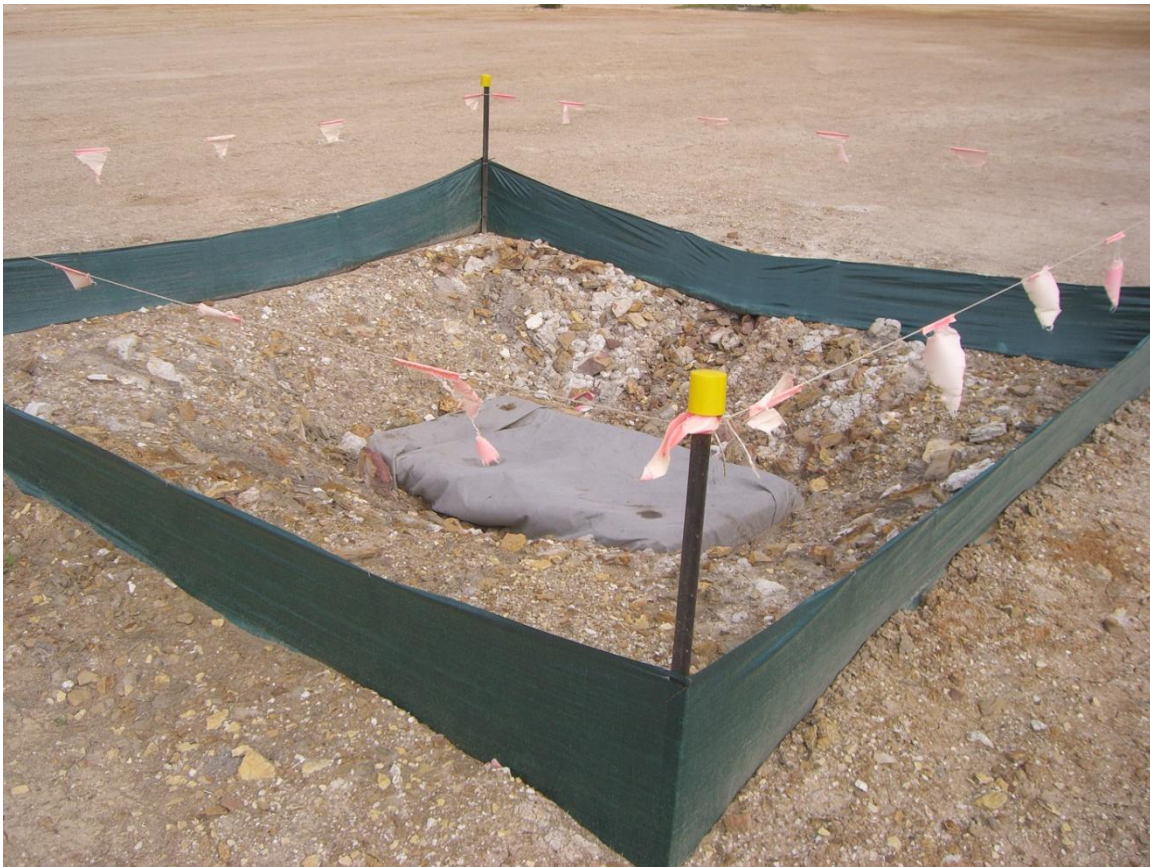
Figure 1 Sediment & erosion controls around stormwater inlet at ILC Site
