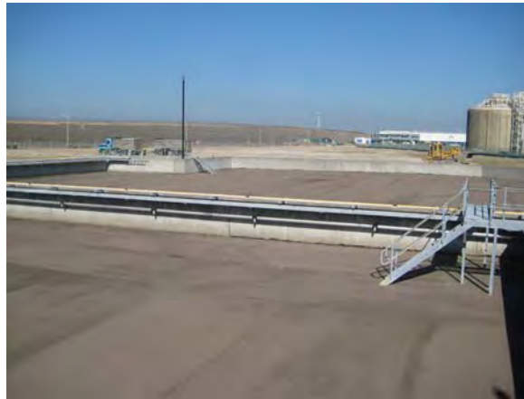
Picture 3 – Existing bunded areas to contain the two proposed tanks
