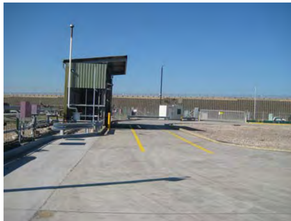
Picture 5 – Entry gate with existing loading/unloading facilities
