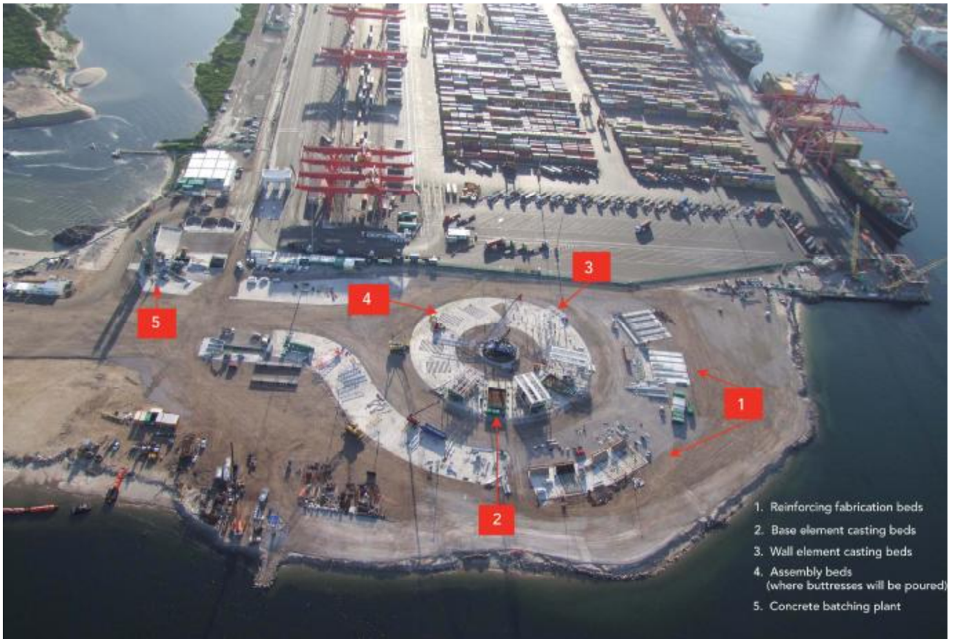
Figure 2. Counterfort precast yard
